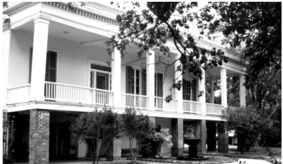
A typical "up river" Anglo American plantation-style home, the Thomas Toby house, sits on raised piers to help protect it from flooding and dampness that caused rot. Toby was a wheelwright from Philadelphia.
